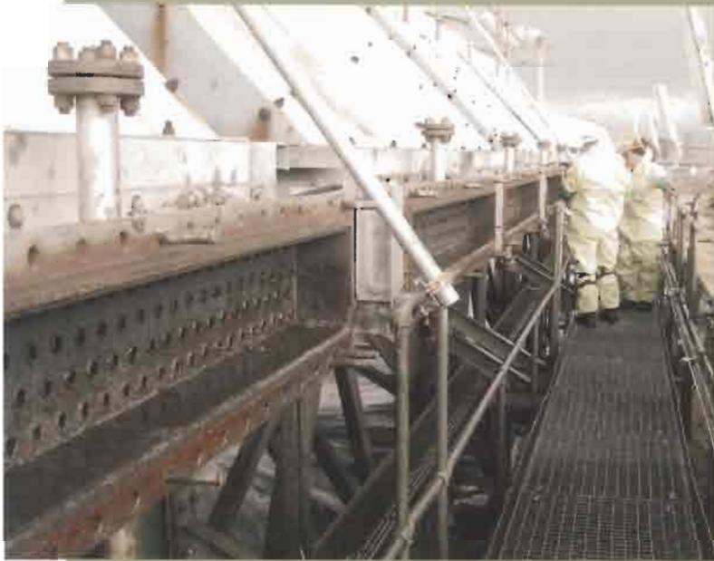
FIG. 7 REFINERY AIR-COOLER BUNDLES
